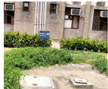
Rainwater harvesting pit
