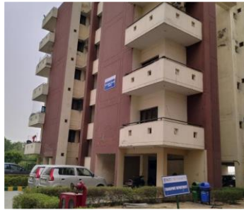
Well ventilated building
