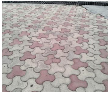
Paving stone installed in campus
