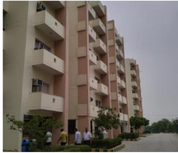
Well ventilated building
